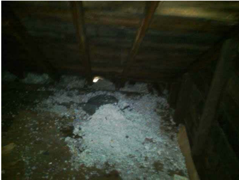
Past staining noted on roof sheathing. Signs of past fire - charring.
