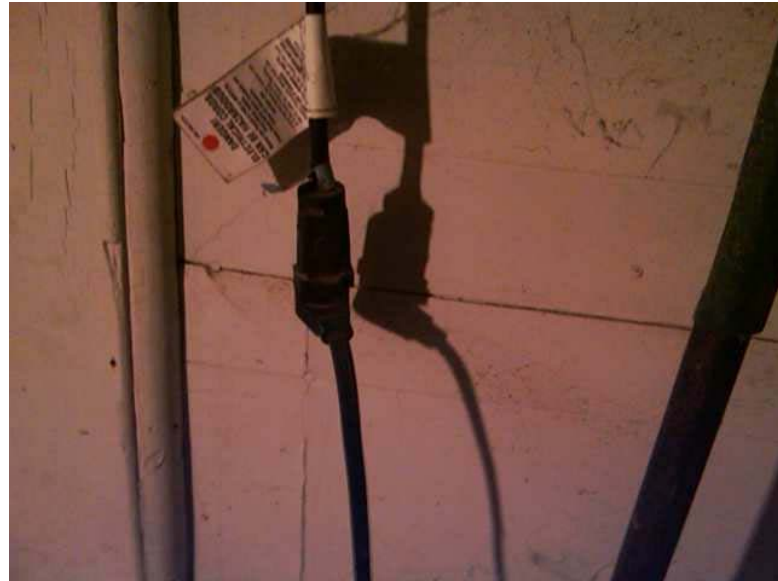
Open junction box(es). Wiring not drilled through joists (run under joists). Extension cords run in lieu of permanent wiring.
