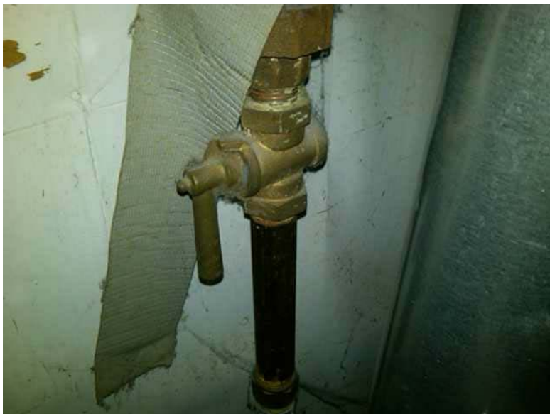
Unapproved gas valves at dryer - Recommend changing to an approved gas shut off valve at next appliance change out.
