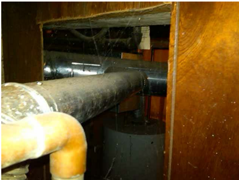
Richmond - downward pitch on vent piping.
