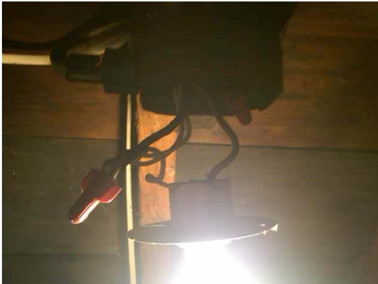
Attic - light hanging by wires.
