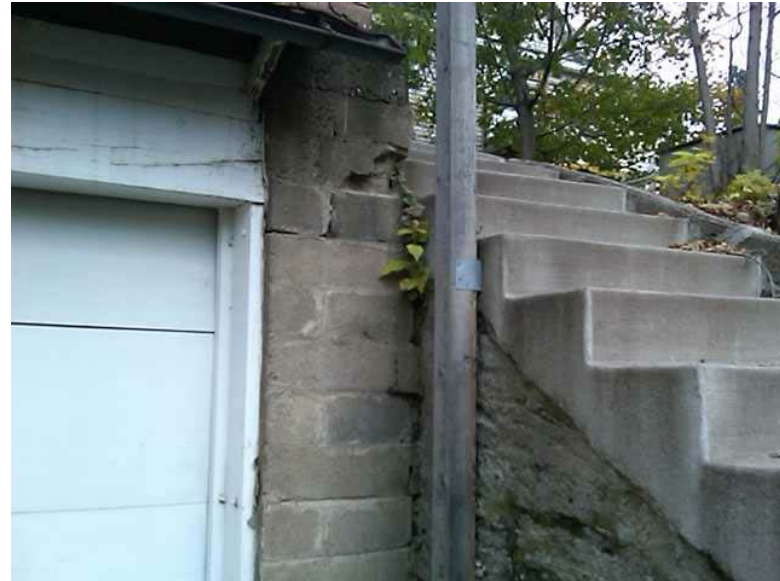
Cracks and past staining on wall components. Decayed shingles and wood on garage exterior. Signs of past moisture on interior garage masonry walls due to poor grade.
