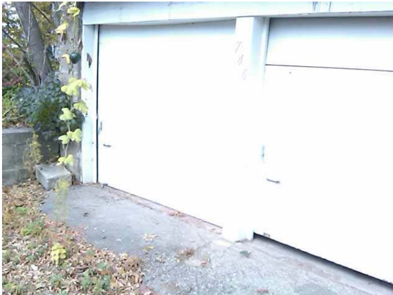
Old weather door panels. East door does not close properly.
