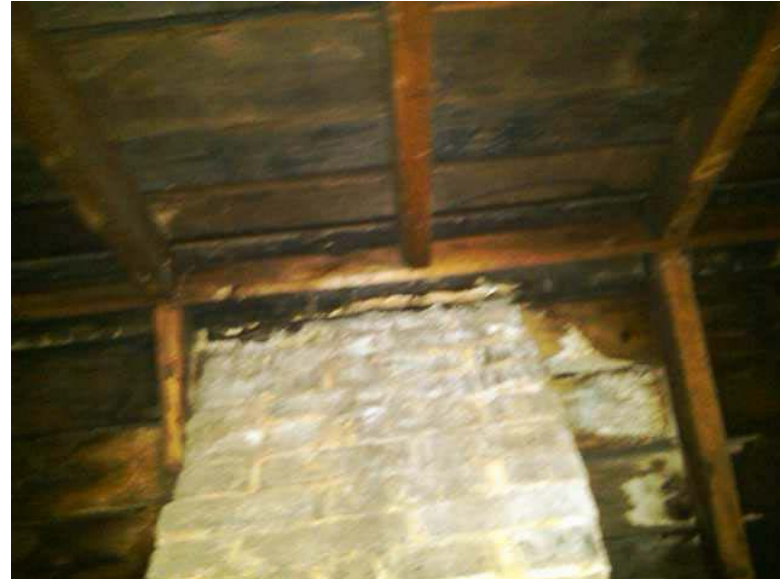
Past stains noted around chimney hole on sheathing and wood members.
