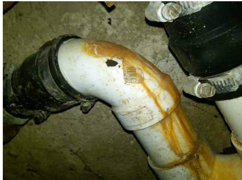
Unable to view all vent and drain piping for basement fixtures due to finished surfaces. Corroded joints. Long trap weir at laundry tub, Improper mission coupling - (lacks a stainless steel collar) at waste assembly.
