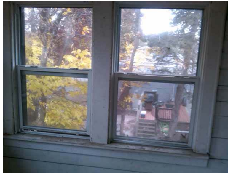
Weathered windows. Damaged screening.
