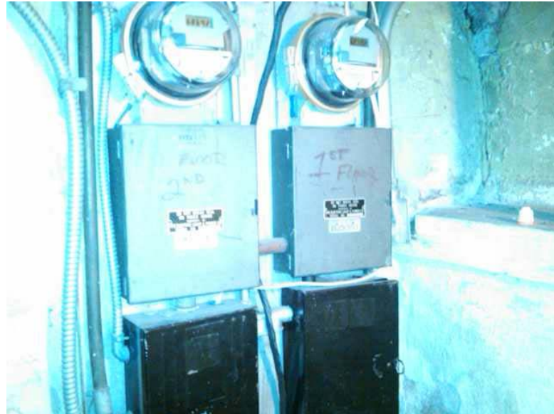
Some circuits not indexed - recommend checking all indexing.
