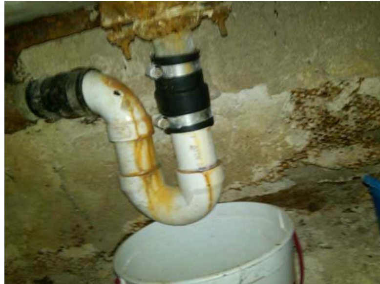
Unable to view all vent and drain piping for basement fixtures due to finished surfaces. Corroded joints. Long trap weir at laundry tub, Improper mission coupling - (lacks a stainless steel collar) at waste assembly.
