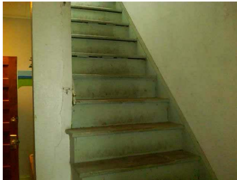
Upper Unit rear staircase - sloped and settled staircase/structure, Lacks handrail(s). Headroom less than 6'8" high. Improper stair rise. Improper stair run. Front staircase - Lacks handrail(s). No railing/guardrail on open side of staircase. Headroom less than 6'8" high. Attic staircase - Lacks handrail(s). Lacks guardrail(s). Headroom less than 6'8"
