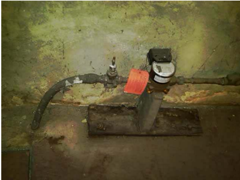
Lead supply line from the street.
