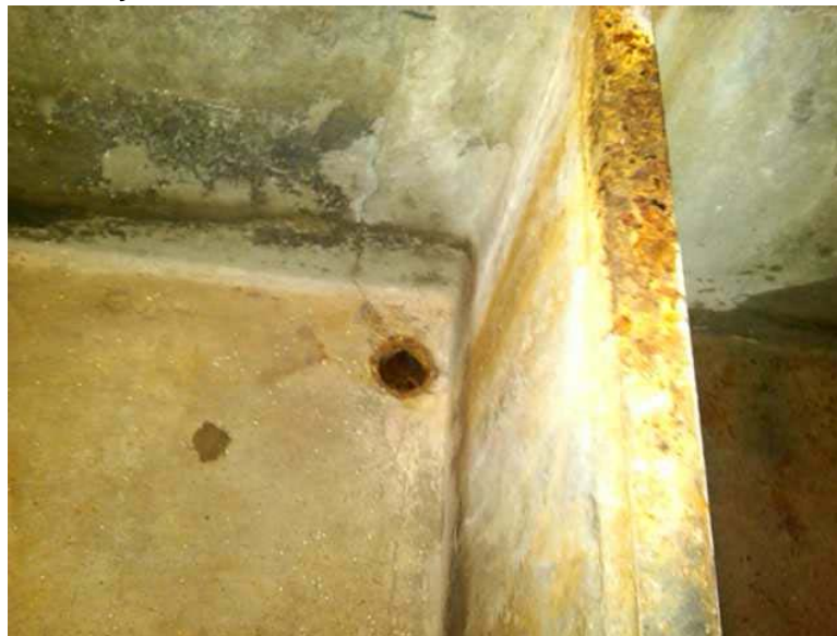
Cracked cast iron laundry tub, Improper drain assembly. No backflow preventer on threaded taps.
