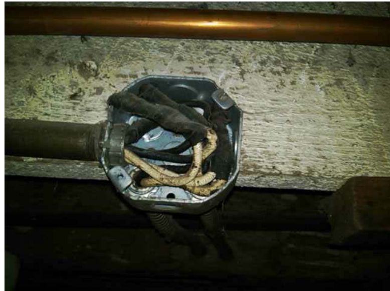
Open junction box(es). Wiring not drilled through joists (run under joists). Extension cords run in lieu of permanent wiring.
