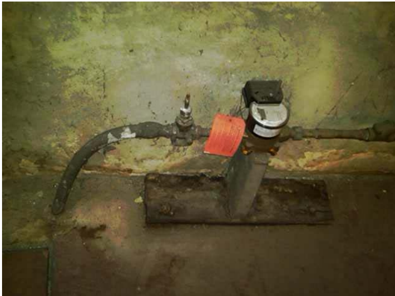
Damaged / missing handle.
