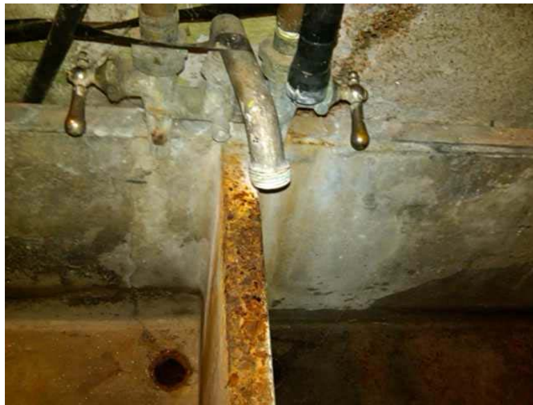
Cracked cast iron laundry tub, Improper drain assembly. No backflow preventer on threaded taps.
