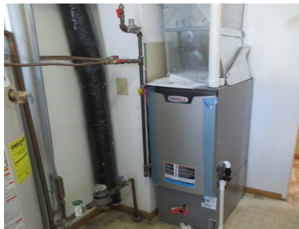
PIC 42) View of New Furnace Installation
