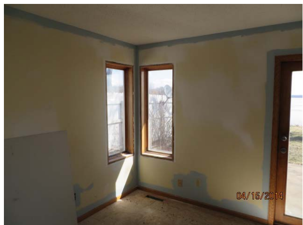
PIC 18) View of demo / drywall repairs
