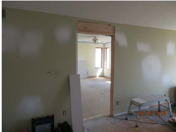
PIC 1) View of Framing/demo/drywall repairs
