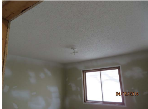
PIC 32) View of demo / drywall repairs
