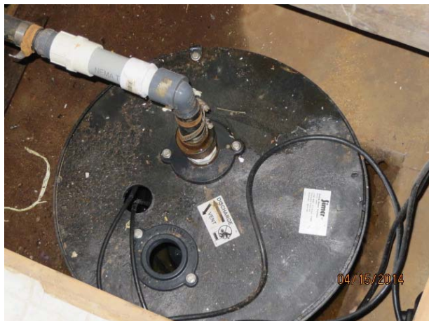
PIC 41) View of New sump/pump-change order.
